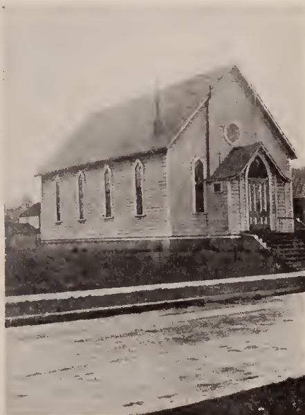
THE FORMER ST. JOHN'S CHURCH, PORTLAND, ORE., TYPICAL OF EVANGELICAL AND REFORMED CHURCHES IN THE PACIFIC NORTHWEST IN THE EARLIER PERIOD OF THEIR WORK
